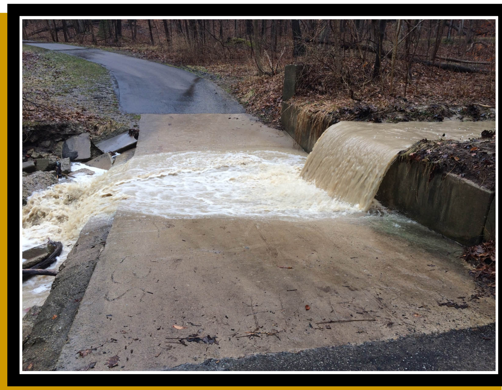
Overflowing weir (left)
